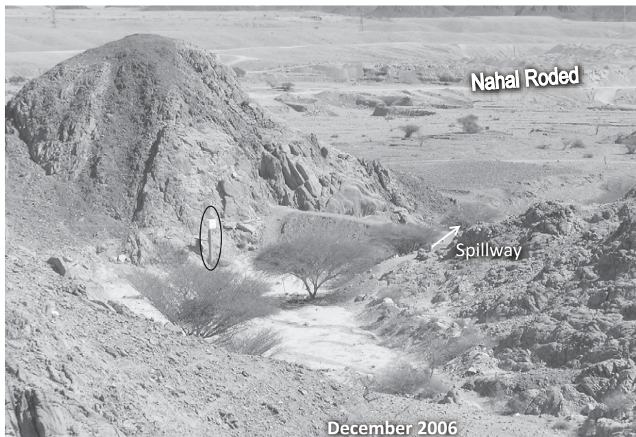
Figure 3. The earth dam and reservoir constructed in 1977 to accumulate all suspended and bed-load sediments before storm flows exited the basin. All the earth material is from downstream of dam (i.e., without digging in the reservoir area). For scale: the gauge station (circled in black) is ~3.5 m tall. The apex of the late Pleistocene alluvial fan of Nahal Yael is seen with desert pavement surface just ~100 m downstream of the reservoir before the confluence with Nahal Roded (Fig. 1C)
